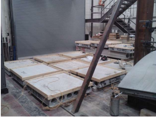
(a) Before casting the topping.
