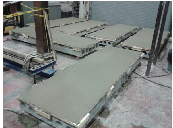
(d) After casting the topping (2 nd shipment).
