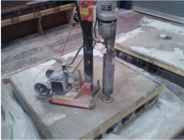
(a) Core drilling.
