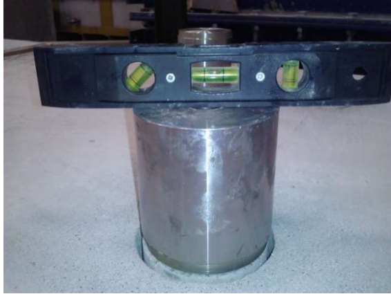
(a) Bonding of the steel disk using epoxy.
