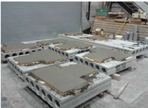
(e) After casting the topping (4 th shipment).
