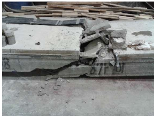
(e) FMB2-3 (flexural shear failure).
