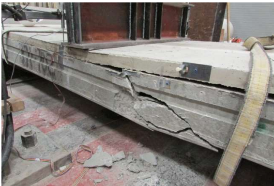
(c) FMB2-1 (flexural shear failure).
