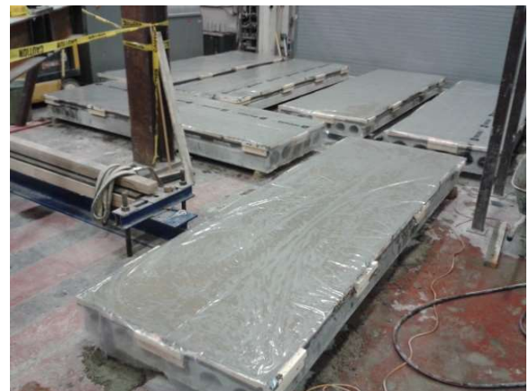
(f) Curing of the concrete topping.
