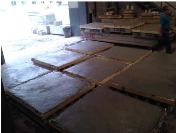
(c) After casting the topping (1 st shipment).
