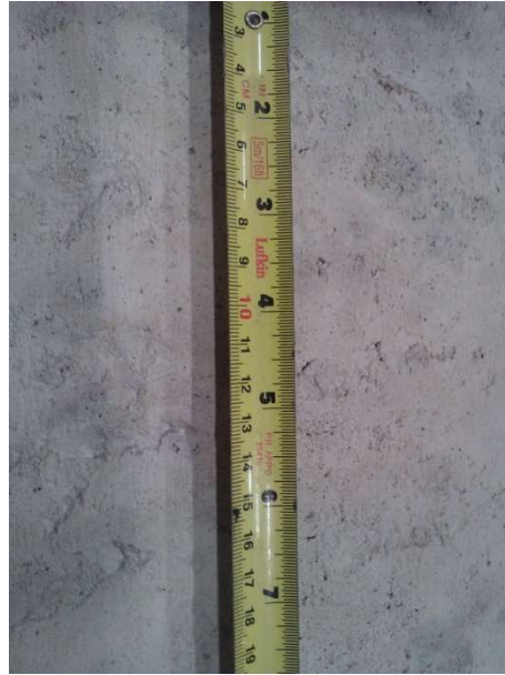
Fig. 1: Typical machine cast finish.
